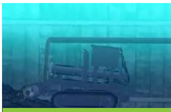
Robotic Sludge Removal In Cooling Tower Basins
