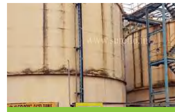
Robotic Phosphoric Tank Sludge Removal
