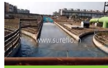
Online Robotic Forebay Cleaning In Power Plants
